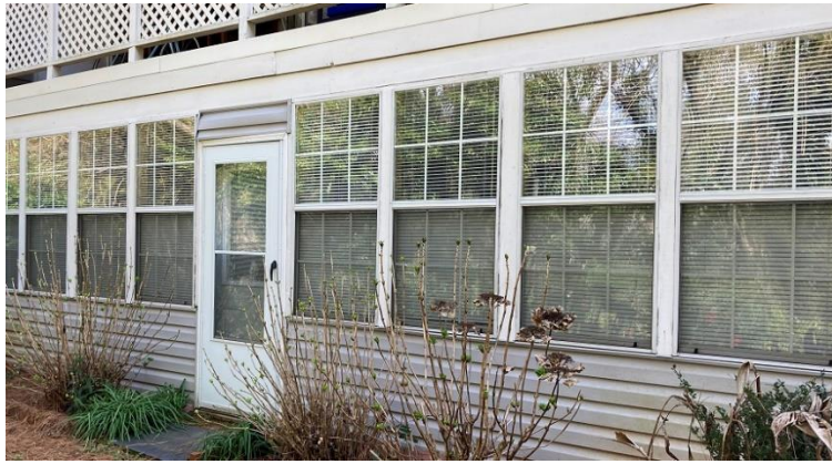
Long Porch With 8 Windows
