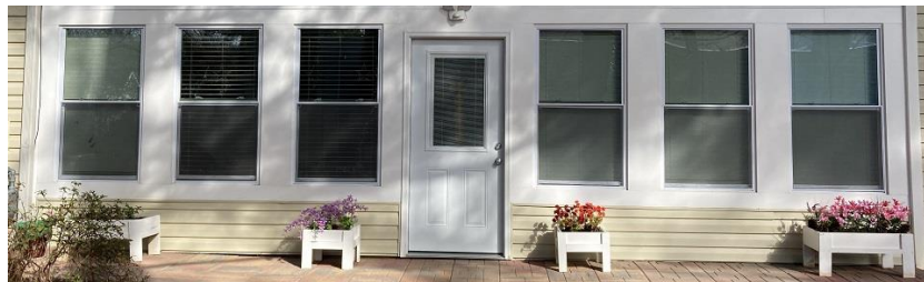
Long Porch With 6 Windows
