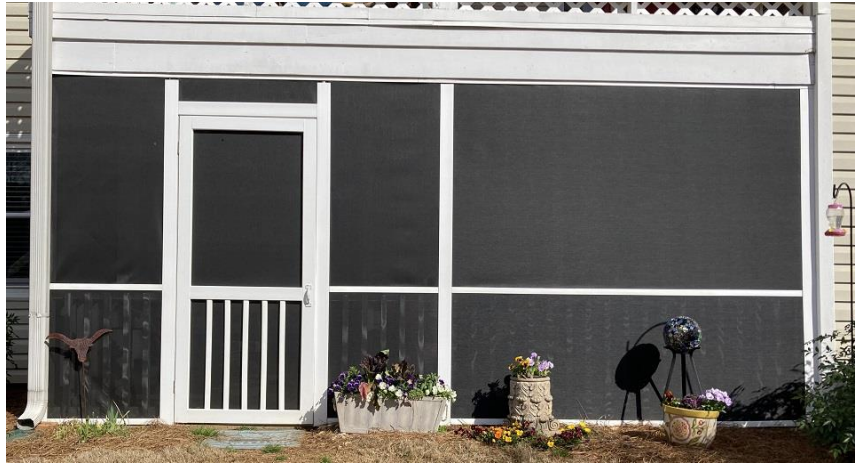
Screened Porch With Balusters
